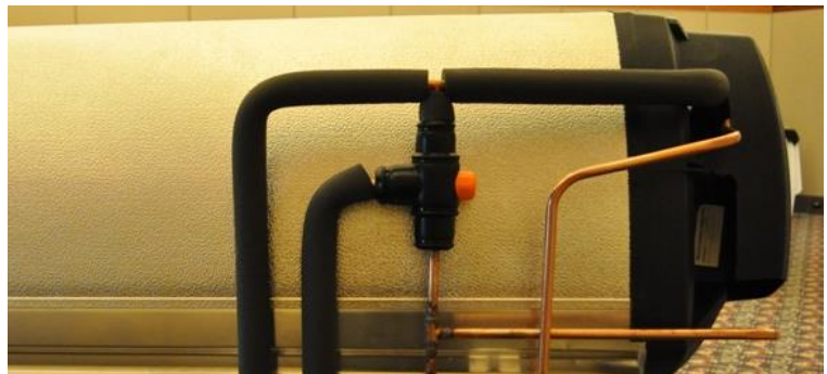
Installation of Pipe Shroud Cover without a HartStat Over Temperature Protection System
